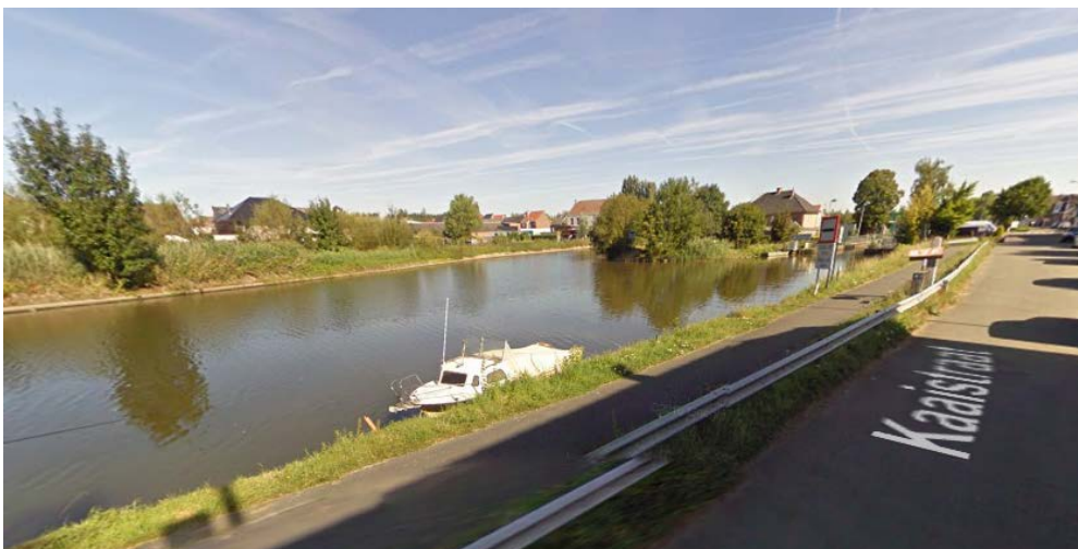
Figure 9 the embankment of the Dender River. Invalid source specified.
