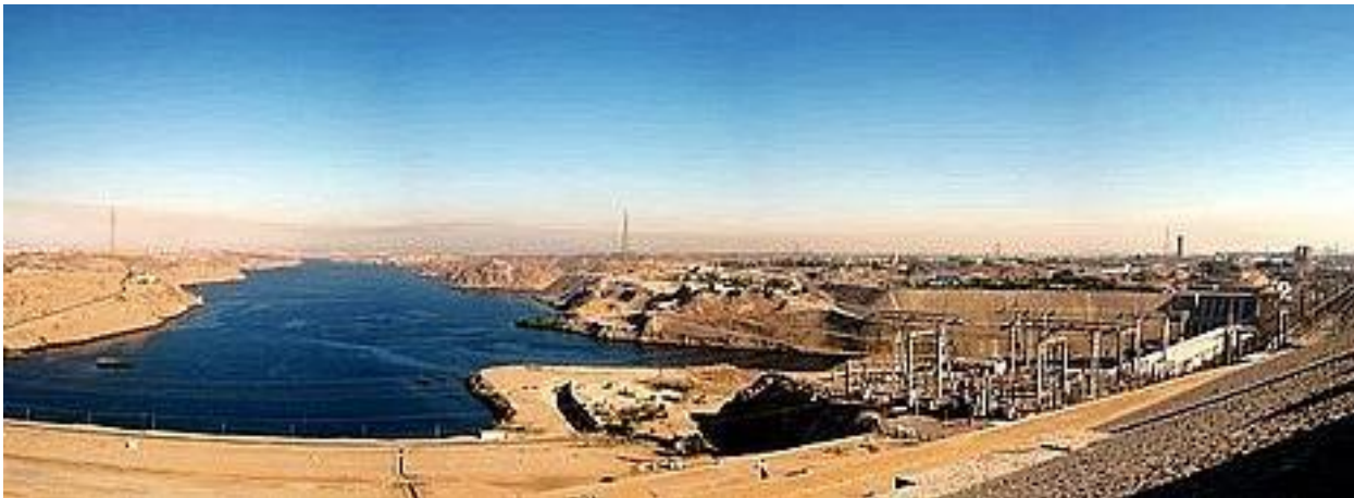
Aswan Dam – Egypt
