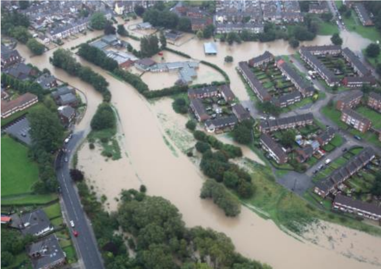
Photo 1: Flooding event, September 2012
